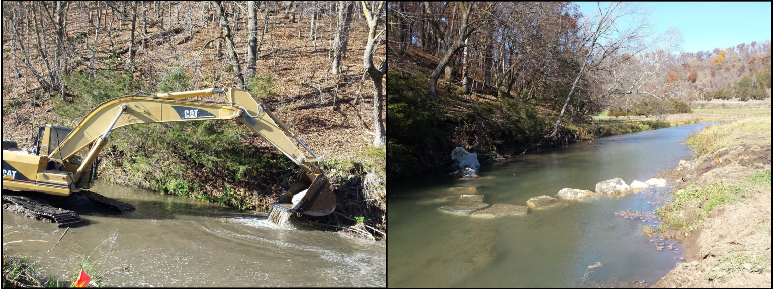
Boulder weir installation on Patterson Creek.
