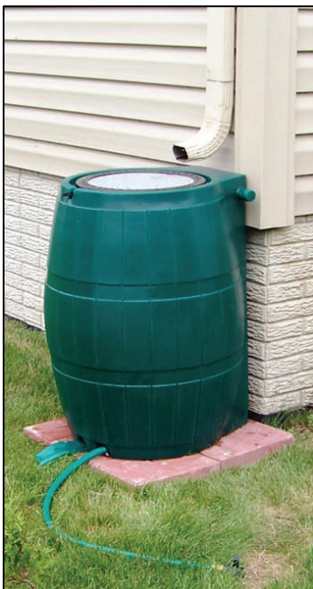
Rain barrel in the Indian Springs Pond Watershed.
